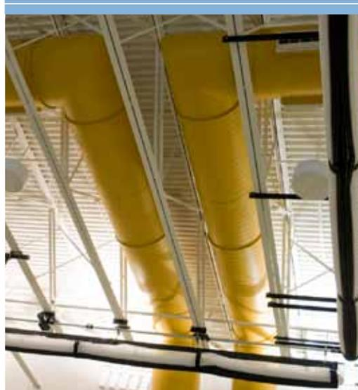
The gymnasium specs called for dual-wall round ducts made of galvalneel.
